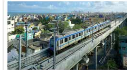
The construction work on the 11.6 km long stretch between Puzhuvhakkam and Sholinganallur begins in Chennai. (Photo credit: Chennai Metro Rail/Representational)
