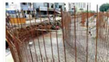
The major stream set to restore the original stream route.
