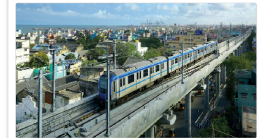
The construction work on the 11.6 km long stretch between Puzhuthivakkam and Sholinganallur begins in Chennai. (Picture credits: Chennai Metro Rail/Kaprasartatana)
